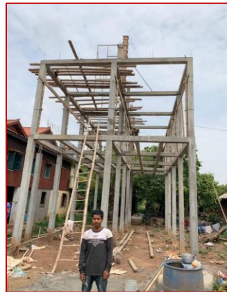
Figure 2: Home under construction
